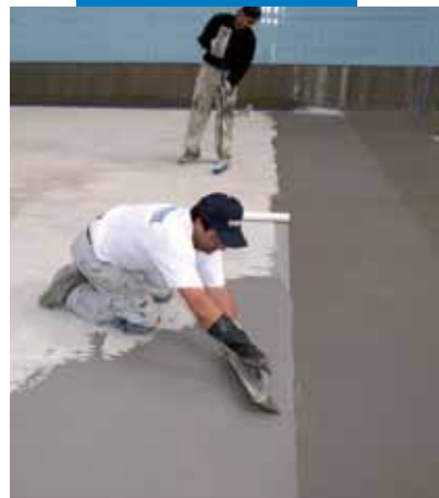
Hydroizolace bazénu Mapelasticem
